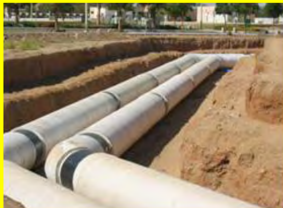
Chiller Cement Lined Piping - KAAU
