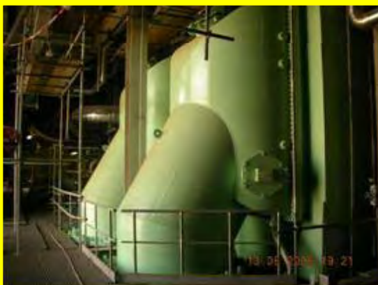
Close Cooling Water Intercooler at Shoaiba Proj.
