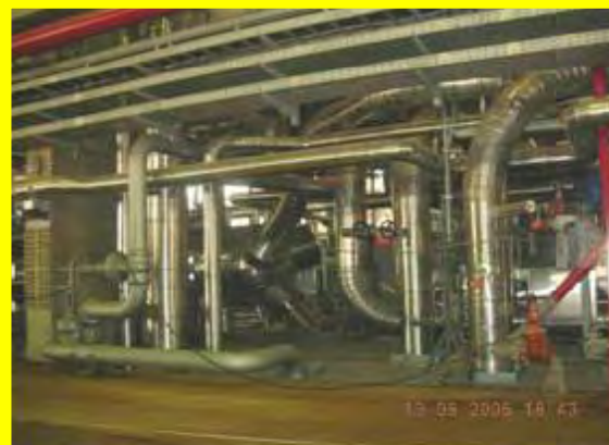
High Pressure Feed Water Pipes Shoaiba 1
