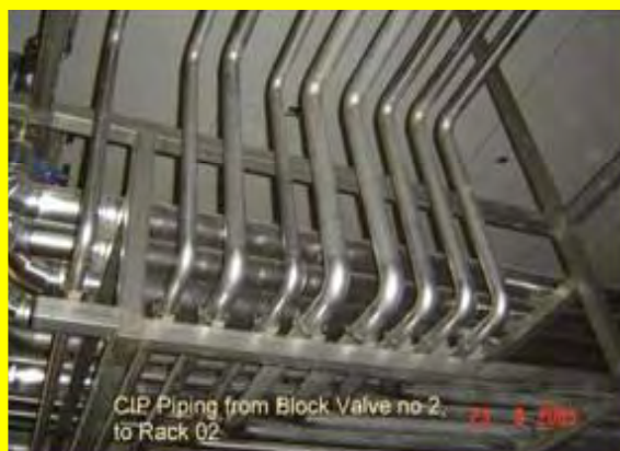
Stainless Steel Pipes – Al Safi Danone
