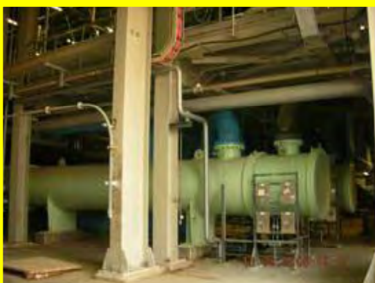
Close Cooling Water Intercooler at Shoaiba Proj.
