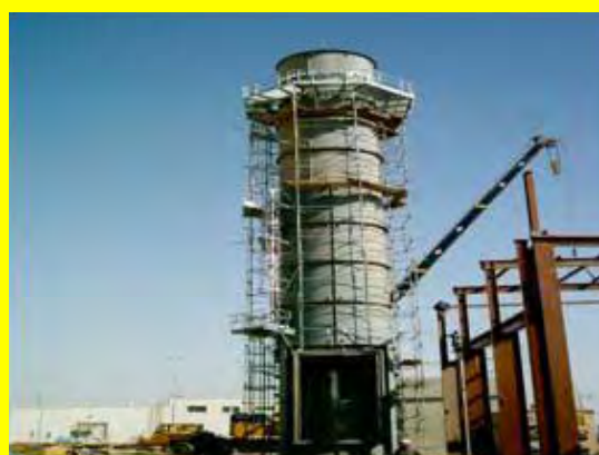
Erection of Stack – PP9 Block E
