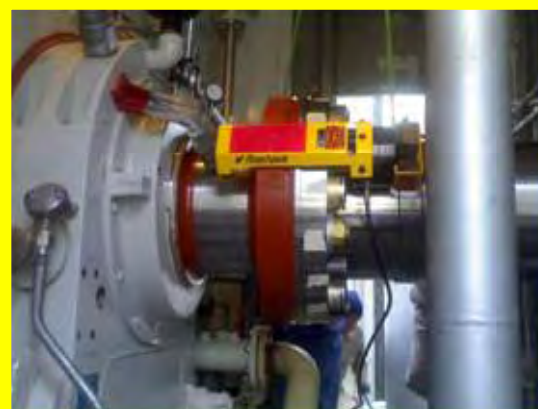
Turbine Alignment at Najran Proj
